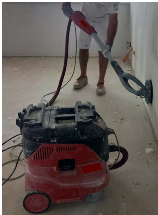
Pictured is a long-neck sander connected to a dust extractor.
